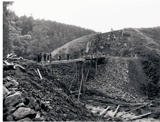
The northern viaduct being built
